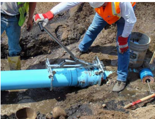
This assembly tool is called the Eagle Claw and is available from Pro Pipe Solutions.
